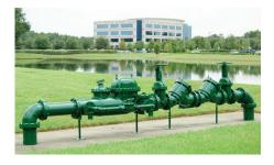
A cross-connection, or backflow prevention device separates drinking water from contaminated water sources. If the flow of water reverses due to decreased water pressure or other disruption in the system, the dirty water can "backflow" into the clean water. Backflow prevention devices create an air-gap between the two sources and help prevent a public health risk, and are often regulated by the health department.
